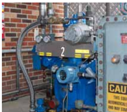
The explosion-proof One Series protecting a natural gas compressor.
