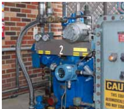
The explosion-proof One Series protecting a natural gas compressor.
